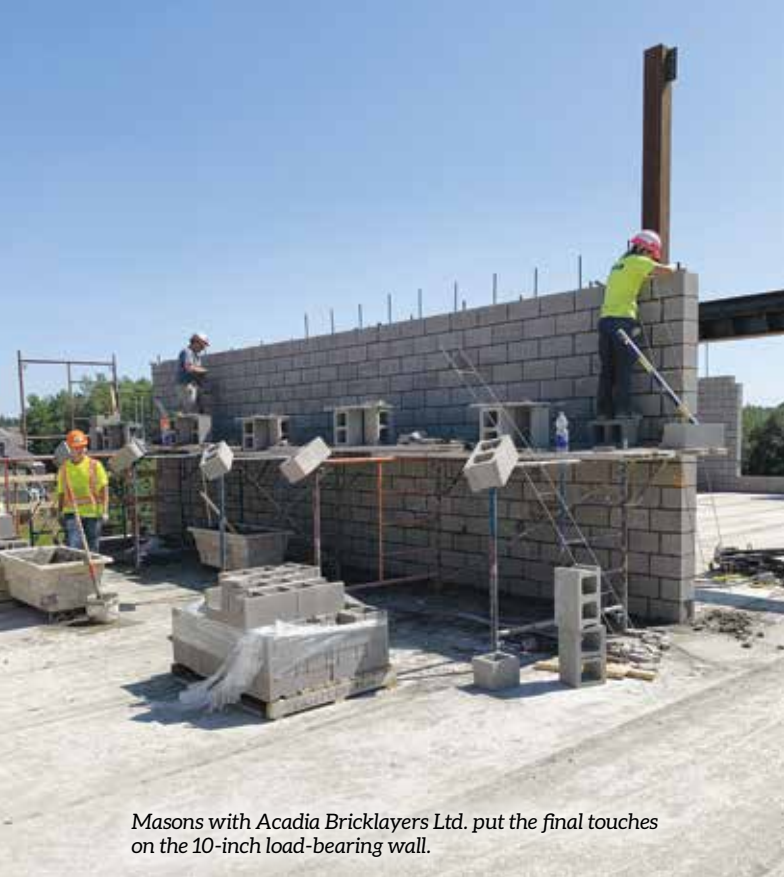
Concrete masonry units (CMUs) ready to be hoisted up and laid in the walls. Job sites with only one trade are clean and organized.
